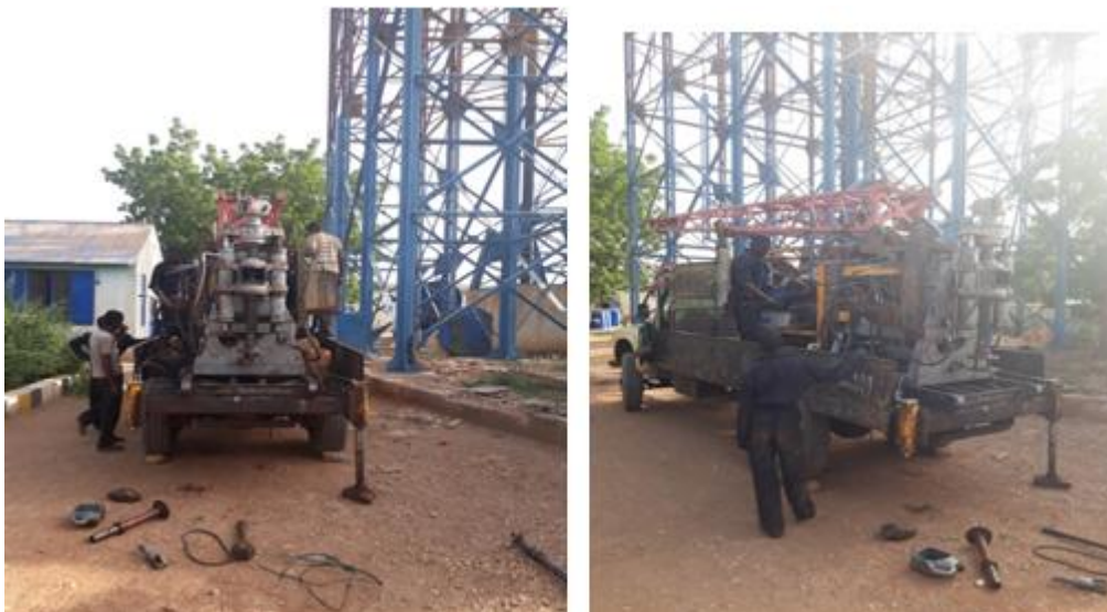
Figure.6 Drilling photo for BAIT ALMAL Station
