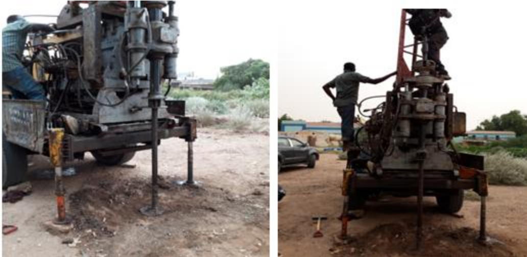
Figure.5 Drilling photo for BURRI Station
