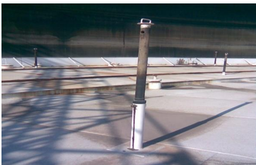
Figure 2- The deck leg of tank
