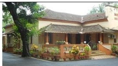
Fig.10 Heritage House Recently Restored
