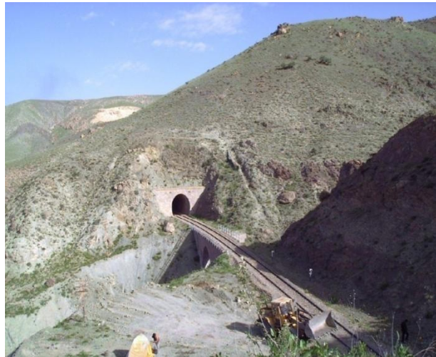
Figure 7-Input and Output trenches of the tunnel
