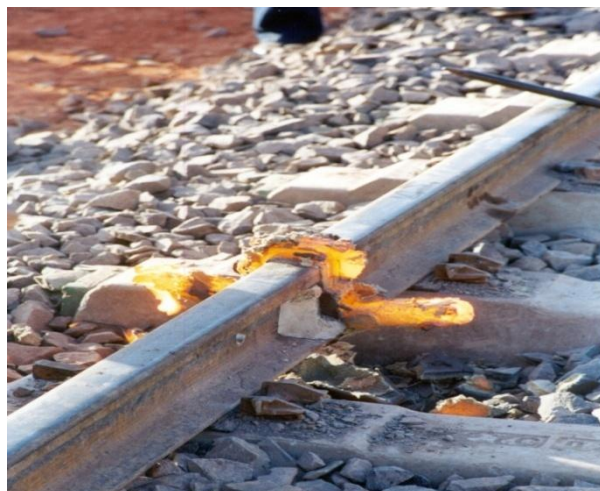
Figure 1 – removing the connection using hermit welding
