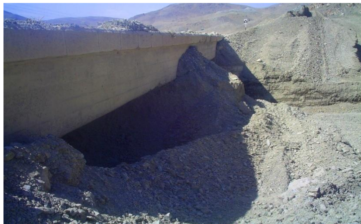
Figure 8 - filling the opening of sediments due to trenching
