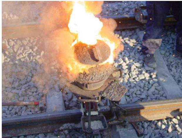
Figure 2– removing the connection using Thermit welding
