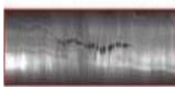
Fig IV: Transverse cracks on observed by magnifying glass
