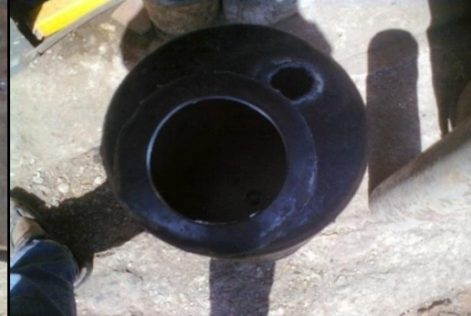
Fig.2.4-Cutting flange for tank
