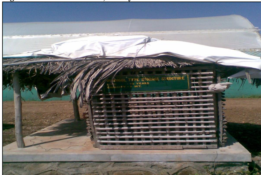
Figure 2: Dindigul onion storage structure
