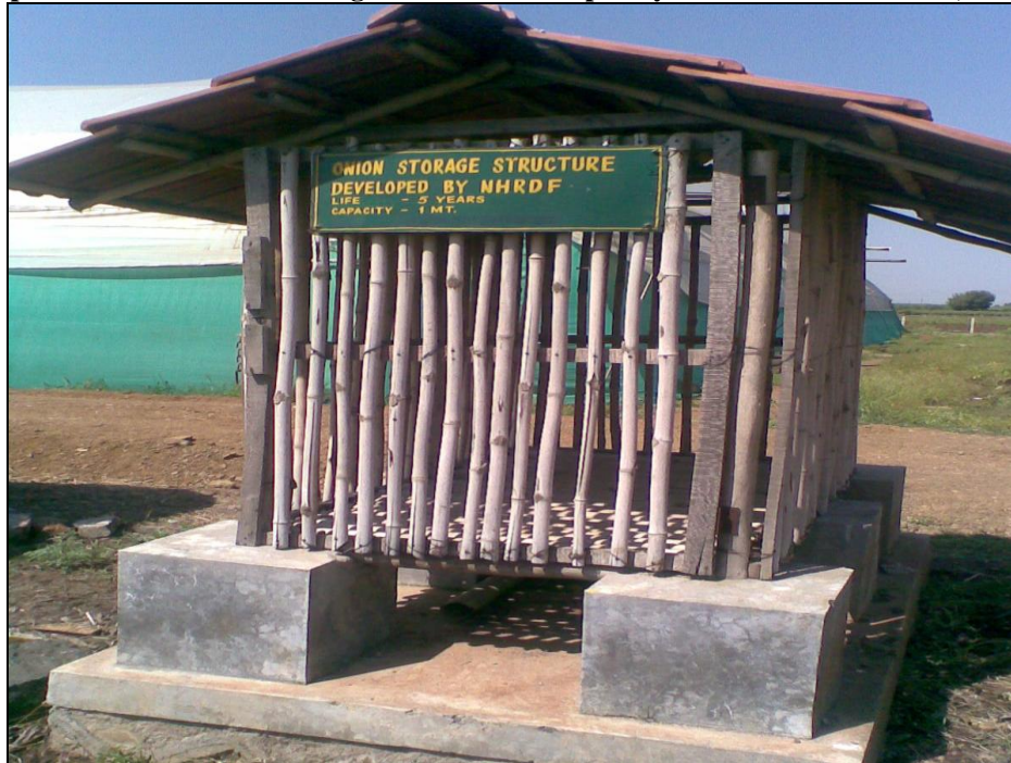
Figure 3: Improved low cost onion storage structure developed by NHRDF
