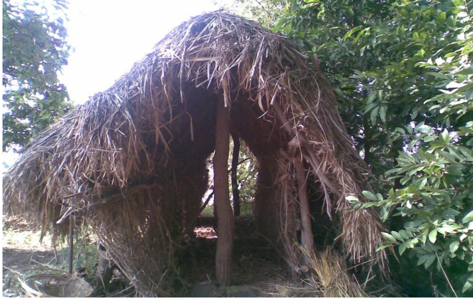
Figure 4: Low cost onion storage structure (Kalwan)
