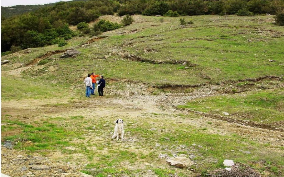
Photo C1: Landslide Area B pigeons (soil material instabilities).
