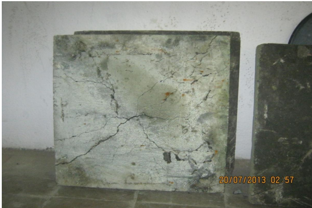
Fig 4.1 Yield line patterns are occurred in slab after application of punching shear.
