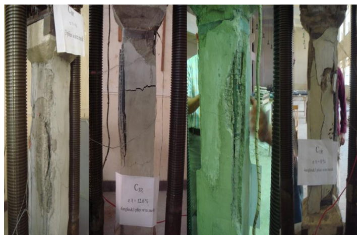
Figure 14: Failure Modes of Strengthened Columns
