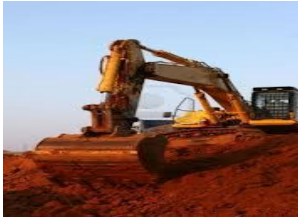
Fig 2: Backhoe Loader in its State of Disrepair (Source: Construction Site, Ilorin)
