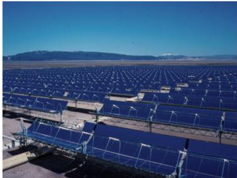
Fig.5 The Solar Bowl above the ground in Auroville, India concentrates sunlight on a movable receiver to produce heat for Electricity
