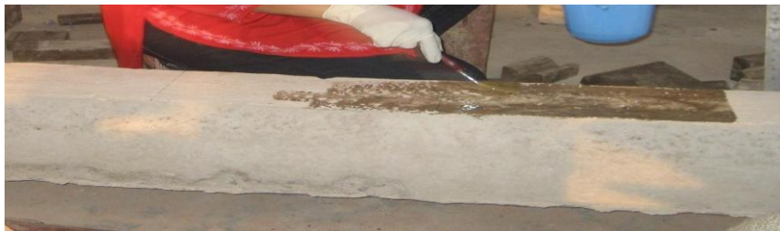
Figure 3.4 Application of epoxy and hardener on the beam
