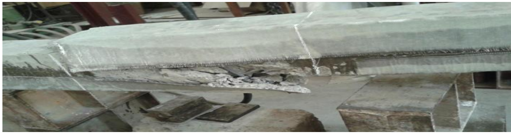
Figure 3.29 Shear crack in the left span
