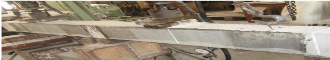
Figure 3.40 Strengthened beam TB3
