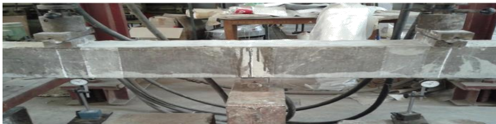
Figure 3.21 Strengthening pattern of beam SB4
