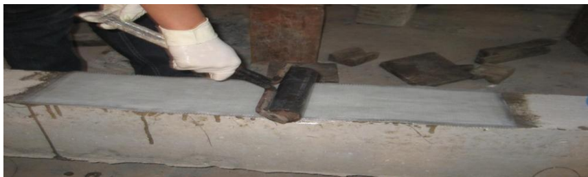
Figure 3.5 Roller used for the removal of air bubble
