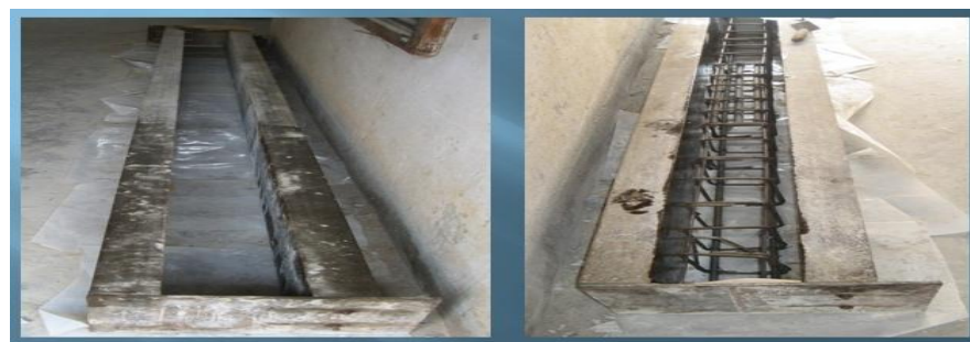
Figure 3.3 Steel Frame Used For Casting of Beam
