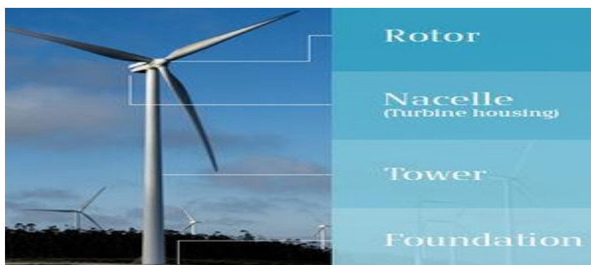
Fig 2.4.1 Parts of HAWT
