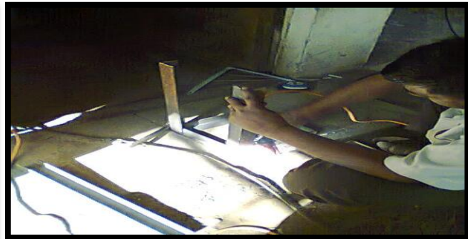
Fig.6(b) Welding operation being performed for Frame
