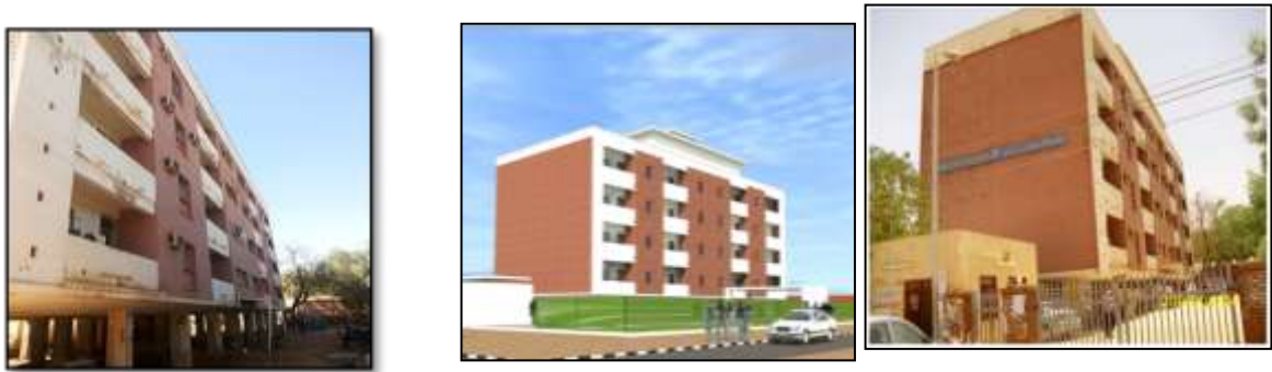
Figure 1. The exterior of building before rehabilitation
