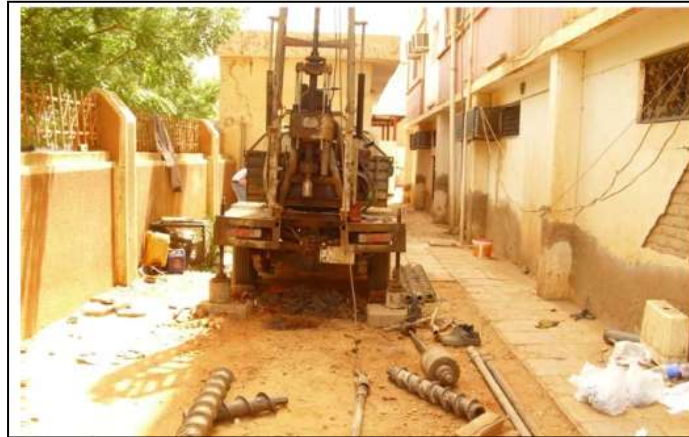
Figure 5 shows the drilling machine to a depth of 10 to 15 meters
