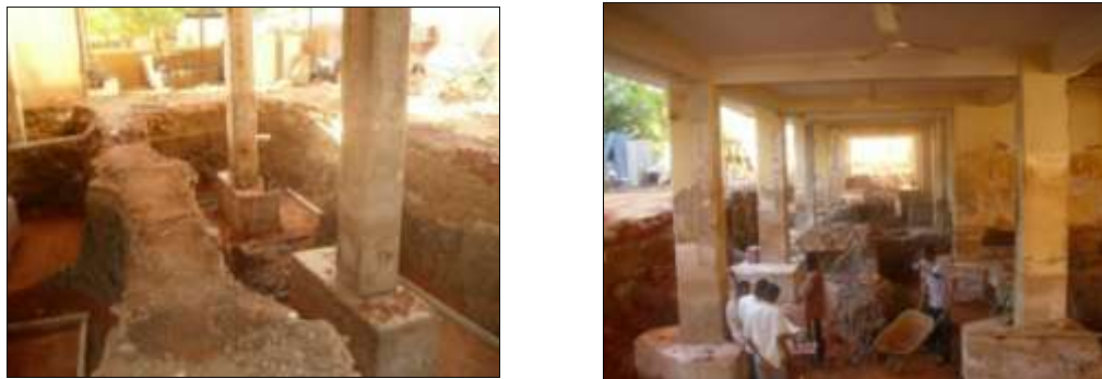
Figure 9 shows the rectangular and triangular pile caps
