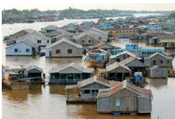
Figure 3: Flooded but Building not rested on the piling system
